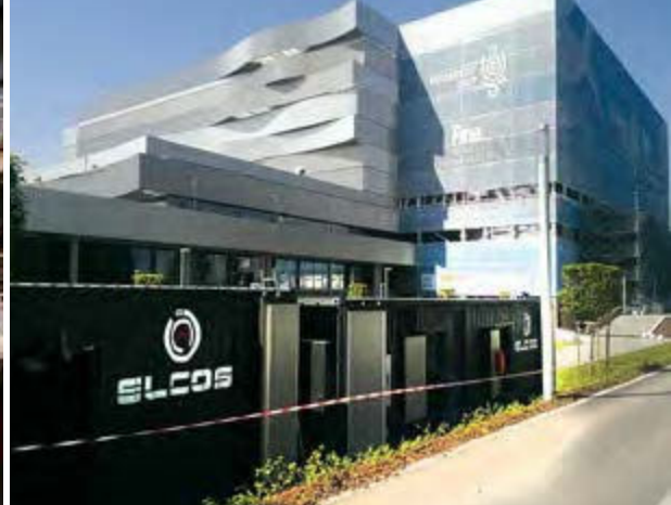
FINA HUNGARY 10 x NO BREAK Power Unit 40 kVA + 8 x NO BREAK Power Unit 20 kVA
