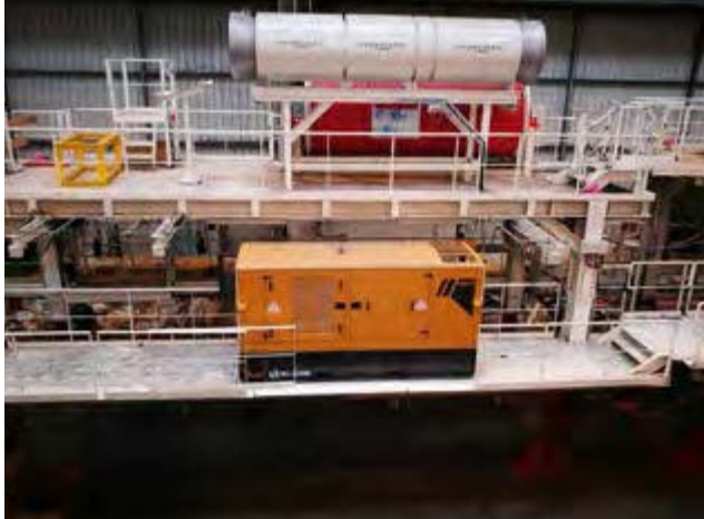
FRANCE - UNDERGROUND WORK 4 X GENSET 225/205 kVA
